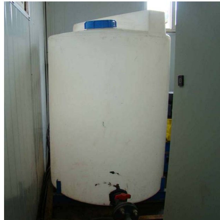
The neutralizer tank
