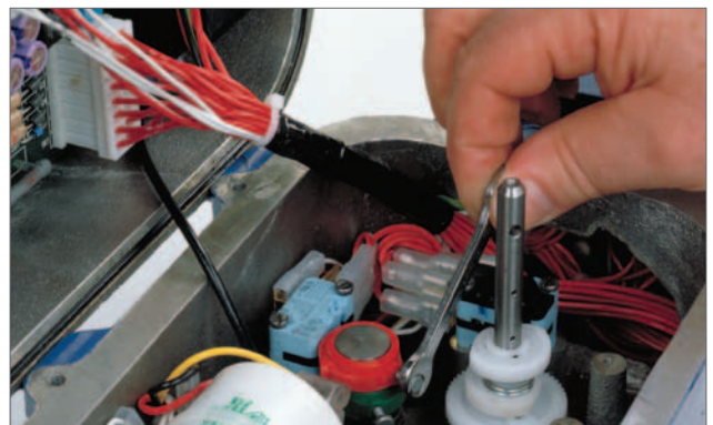
Torque switch setting
