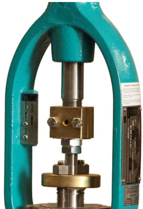
Typical Stem Connection
